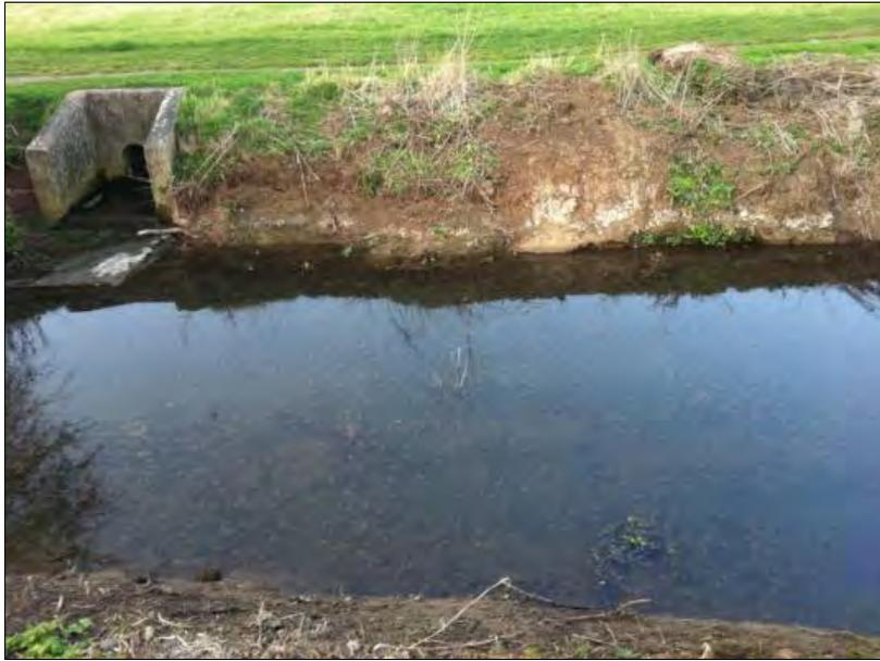
Plate A-1: Further over-widening of channel between sites 2 and 3, combined with bed lowering has resulted in almost no flow velocity (March 2012)
